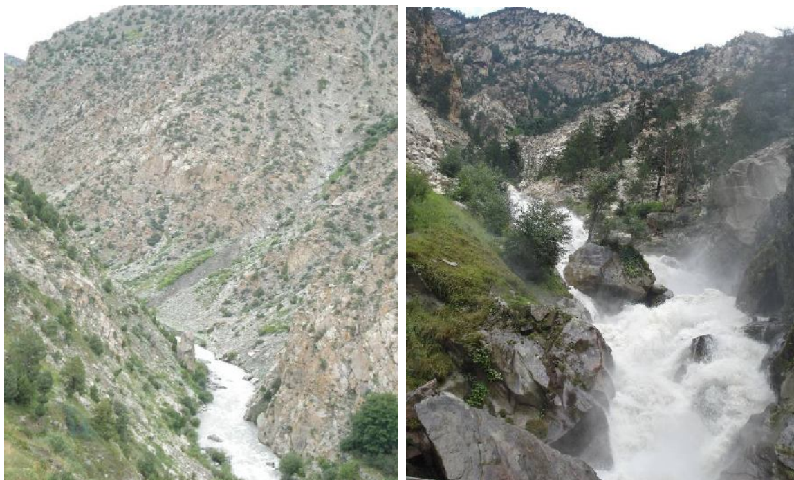
Photo 1 & 2: Kerang stream to be diverted and linked to Kashang streams to generate 243 MW of electricity
