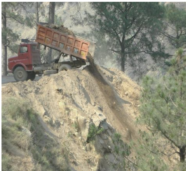
Photo-21& 22: Muck Dumping at Sawra Kuddu project site- violation of clearance conditions
