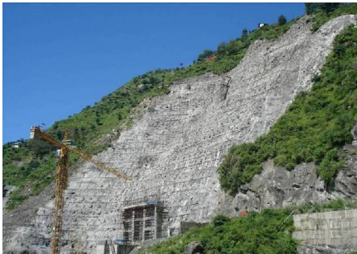
Photo-16: Concretisation of mountain in Parvati-II HEP in Sainj valley
